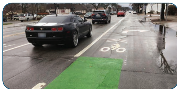
Coolidge during the road diet as a Complete Street with separate areas for vehicles, bicycles and pedestrians.
